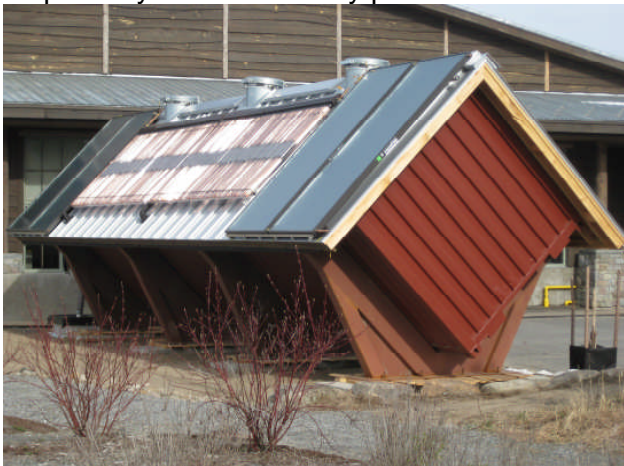
Fig. 4 Pellet storage bin with mounted flat plate and evacuated tube solar thermal collectors.
