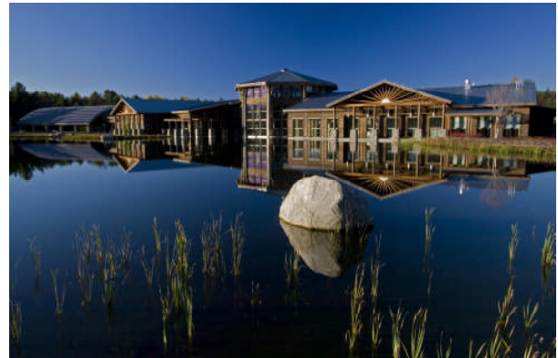
Fig. 1 54,000 ft² Wild Center Building
