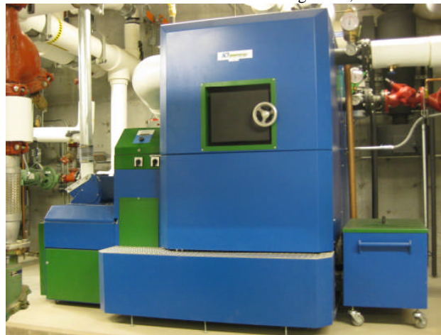
Fig. 2 Front View of ACT Bioenergy Boiler showing combustion chamber and control panel
